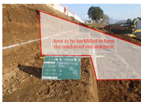
Fig. 6.5 Bench cutting
