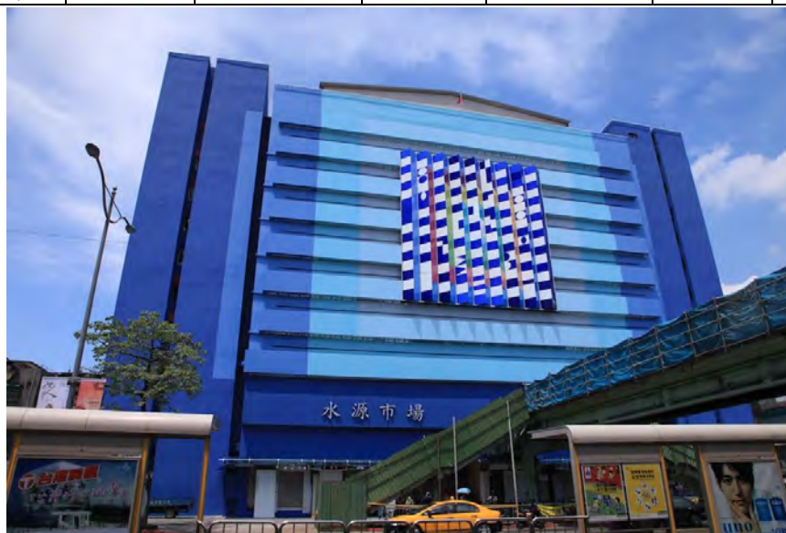
Fig.2 Appearance of Shui Yuan Building
