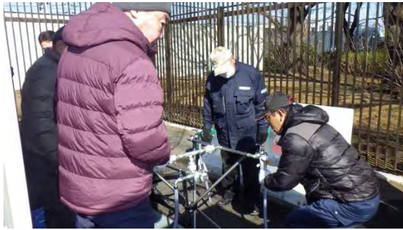
Figure 16. Experience of setting up temporary hydrants
