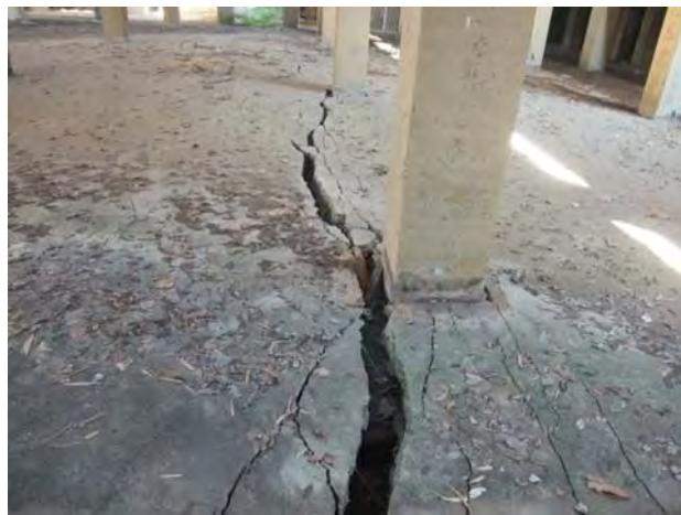
Figure 4 split of bottom slab
