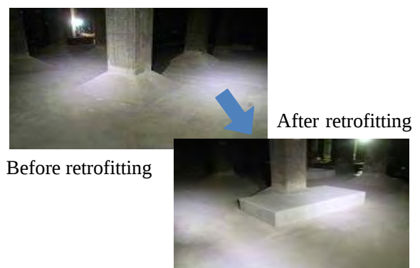
Figure 3. Concrete deck-slab reinforcement
