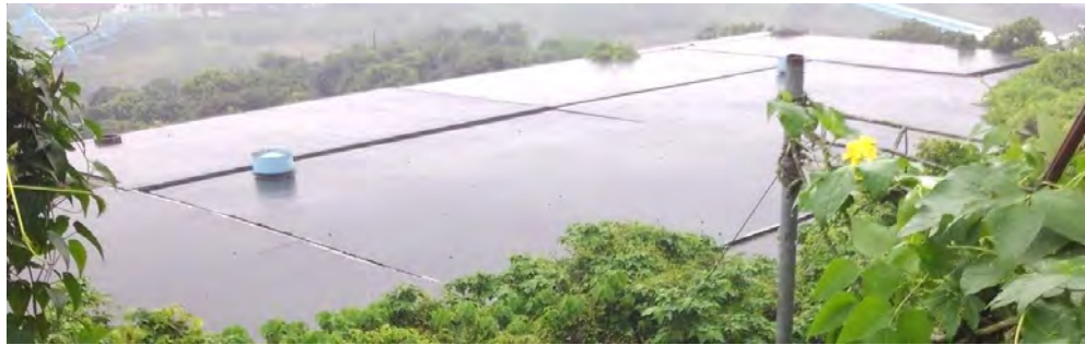
Figure 1 The roof of water tank – the failure of extension joint by expansion
