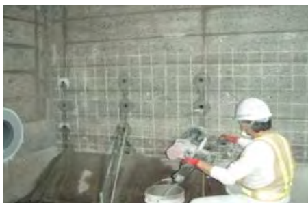
Figure 2. Sidewall boring
