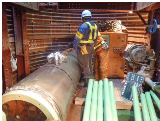
Picture-2: witnessing of pipe jacking work
