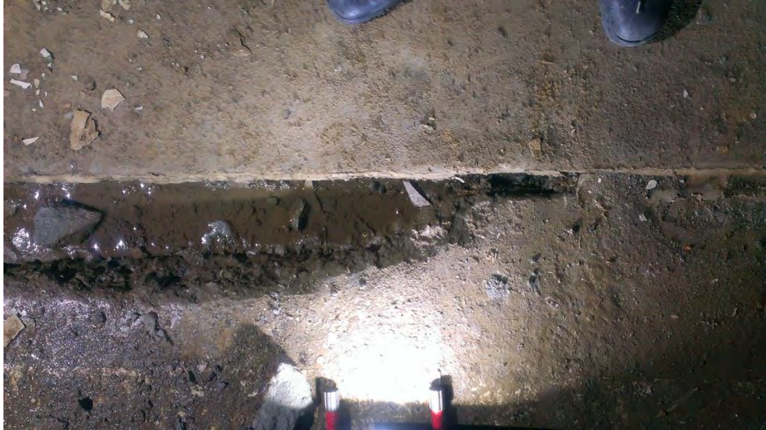
Figure 3 The crack caused by interactional bump of base plate of water tank
