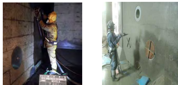
Coating removal Mortar corrosion protection
