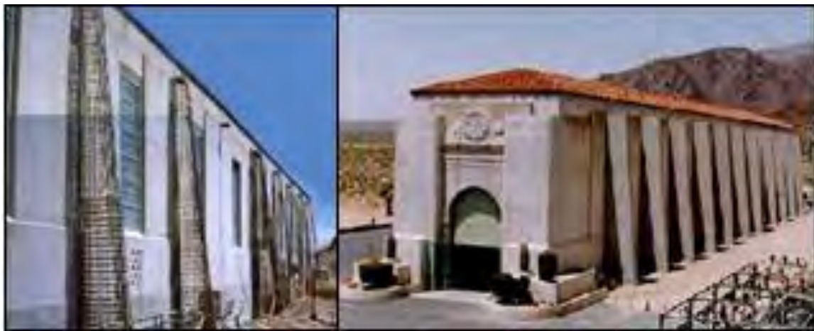
Figure 2: Seismic Upgrade of CRA Pumping Plant
