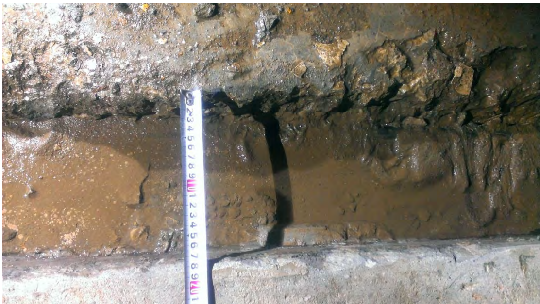
Figure 4 The expansion of the extension joint
